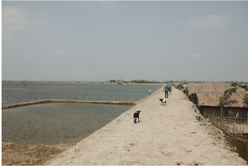
Figure 2. A polder in Khulna, Bangladesh, separates a village (right) from a distributary of the Ganges River (left). Source: Photo by Jonathan Gilligan.
